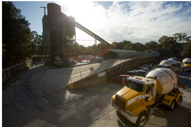
Concrete plant in Alexandria
